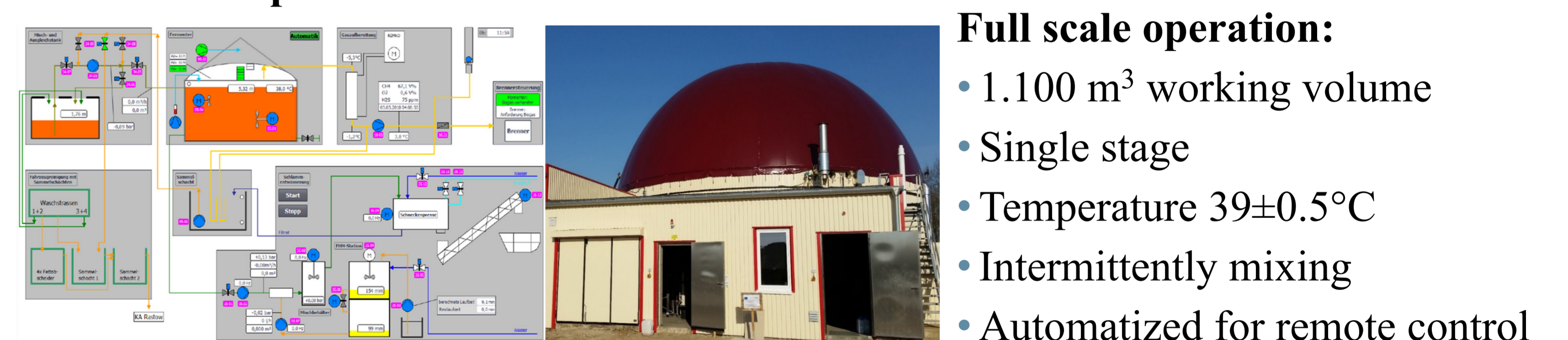
Fig.5: Operation panel of and full-scale biogas plant at TS-Clean, Fahrbinde
